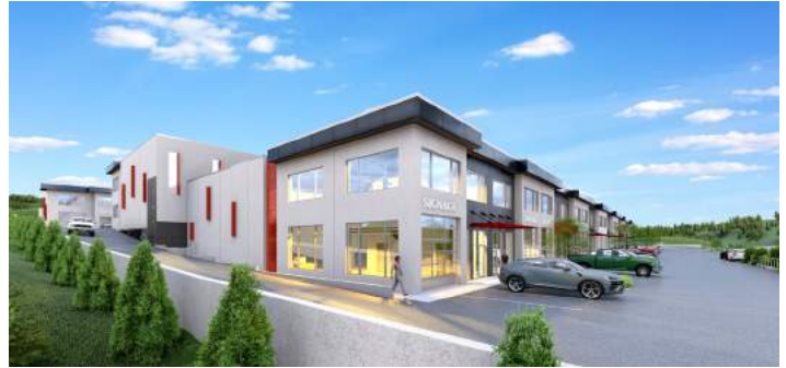
Carrington Industrial Business Park - now Under Construction
